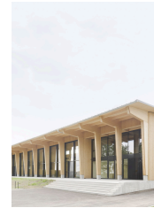
Multi- Purpose Hall by Atelier Kaiser Shen
